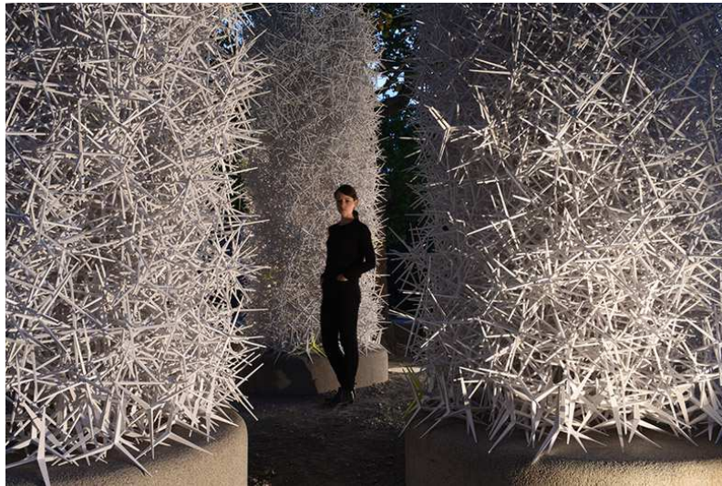
FIGURE 1.8: The ICD Aggregate Pavilion 2015 from the University of Stuttgart. They used 30,000 spiky components and a robot to create a pavilion described as the "first architectural structure realized with a designed granular system".
